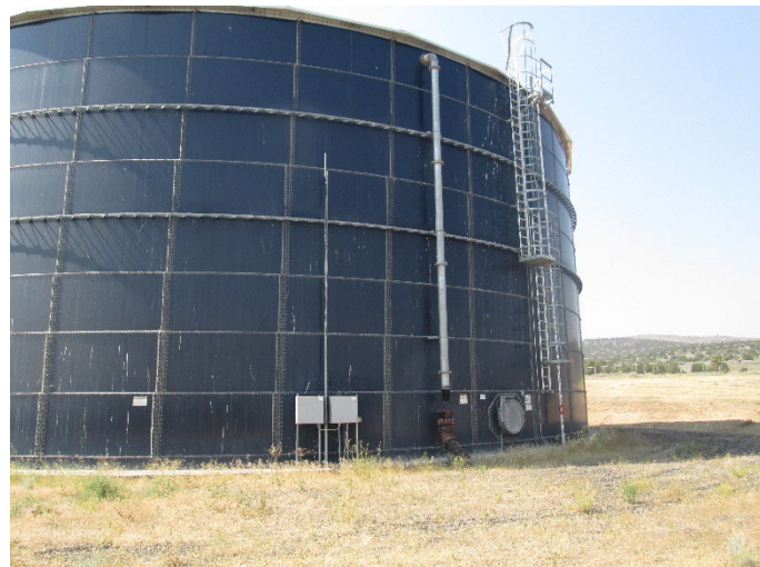
The 2.0 MG glass-fused-to-steel bolted reservoir built in 2002.
