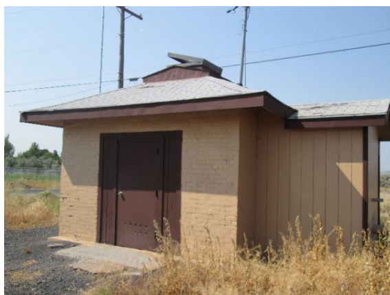
Well No. 1 pump station building.
